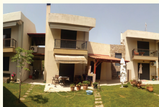
2. KUĆA MARIA GPS N39.99191/E23.98988
