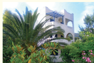
4. KUĆA KALAMITSI STUDIOS GPS N 39.991481/E 23.989227
